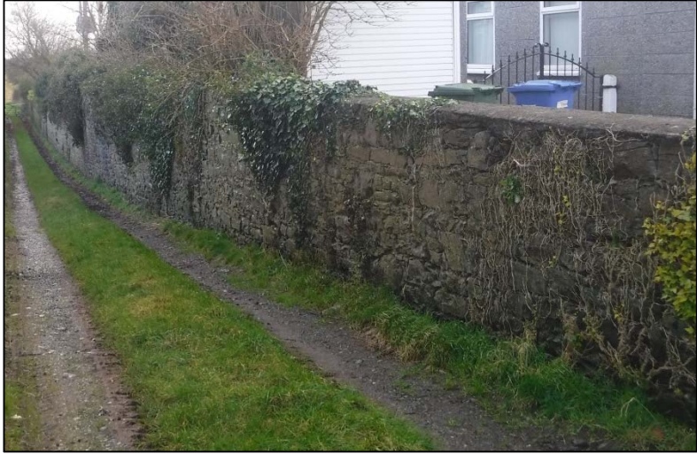
Site CH-2 Eastern perimeter wall to Garda Station
